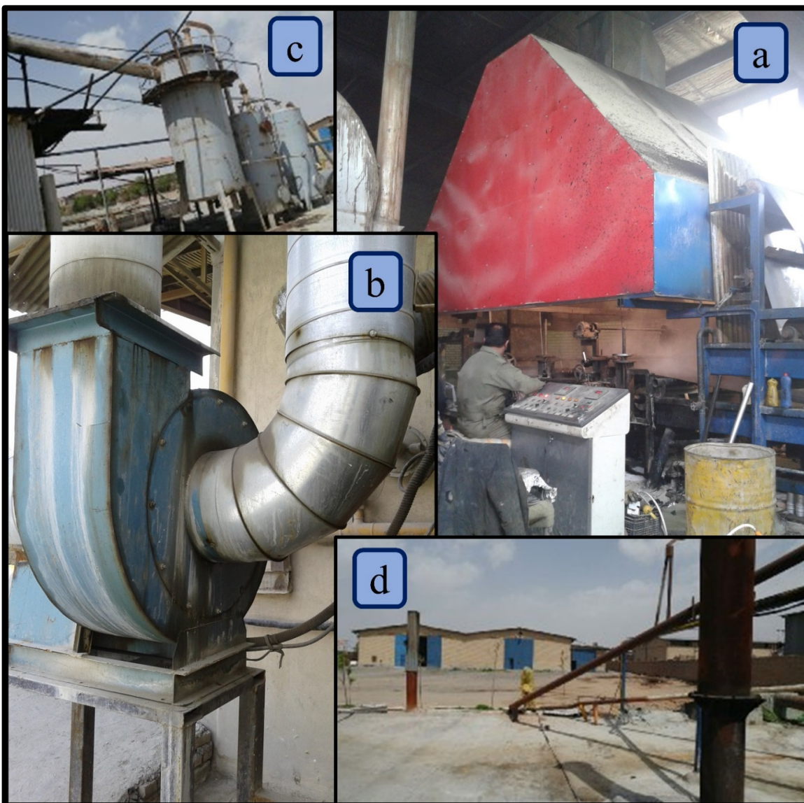
Figure 1. (a) Hood collects gases from the tissue exit from the pond, (b) Indoor gas suction fan, (c) Indoor gas transfer to three-stage scrubber towers, (d) Transfer of gases from scrubber (wet detergent) to re-combustion furnace.
