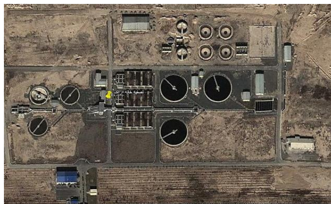
Figure 1. View of AWWTP with its unit processes
